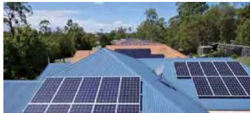
Metal Roof Mounting System
